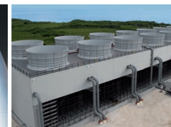
Cooling tower installations
