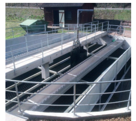
Round tank converted to TUBEdek®
