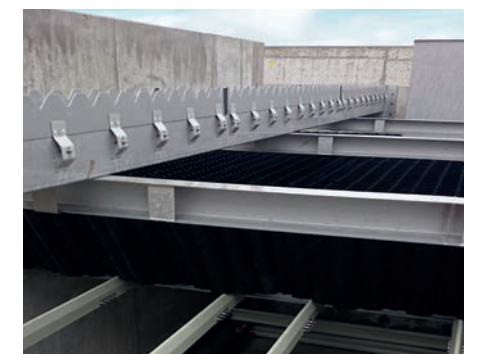
TUBEdek® with support structure and launders
