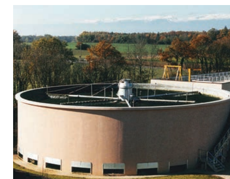
Secondary sedimentation after biological fixed beds – combination of trickling filters and lamella separators
