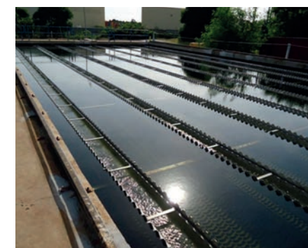
Drinking water plant upgrade
