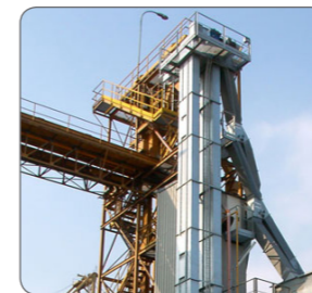
Belt Bucket Elevators
